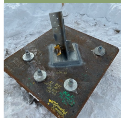
Pile Cap Installation
