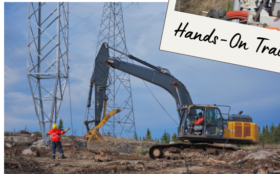
Classroom knowledge and hands-on hours on loaders, excavators, and dozers.
